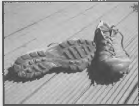
Flyroc 310 after 18 months)
